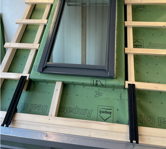
Attach Megasol MATCH Slate hooks according to planning information or individual arrangement.
