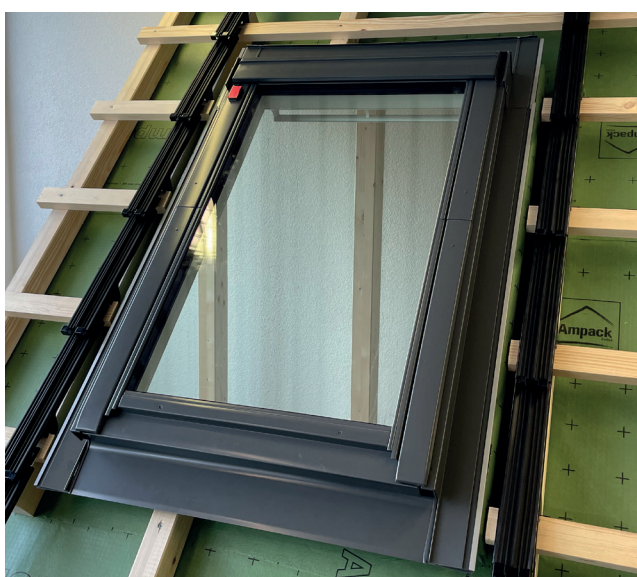
Fully assembled ODL flashing.
