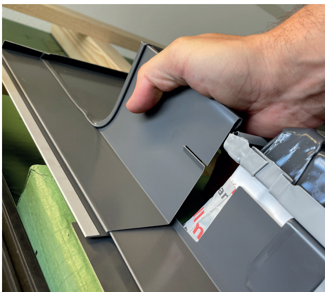
Slide the flashing head piece into the side rebate.
