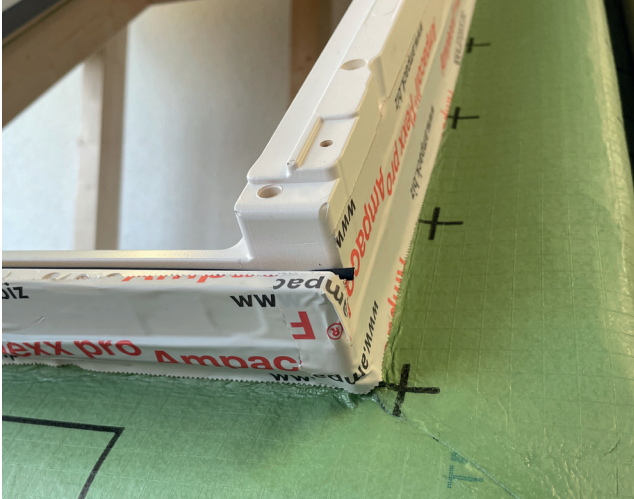
Apply nail sealing tape to the counter bracket (guidelines of the under-roof membrane manufacturer) and install according to the batten plan.
